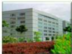
Fuel for Gas District Cooling
